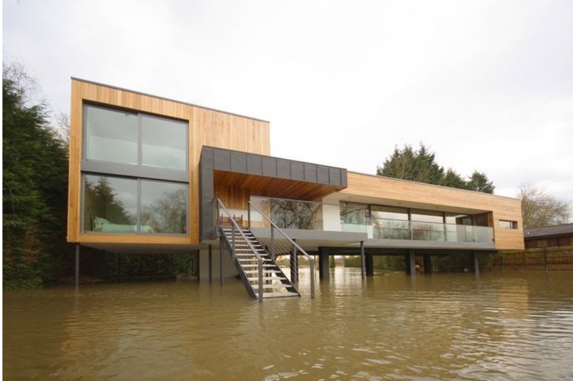
Parday House near Wargrave: a completed home is raised up on a steel frame, above ground level
